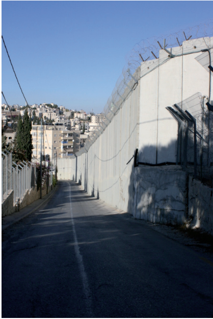
Separation wall, separating Ras Al-Amud from Abu Dis
